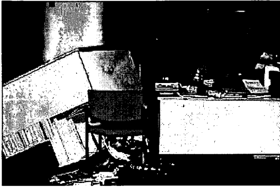
Figure 7. Overturned file cabinet. File cabinets are prone to overturning because of their slenderness, and they are even more vulnerable when unlatched drawers can slide out. This photo of the Santa Clara County Administration Building after the 1984 Morgan Hill Earthquake, shows that desks proportions make them unlikely to overturn and thus they provide good protection against nonstructural damage if occupants are trained to quickly take cover (Photo credit: EERI, Wesley Van Osdol).
