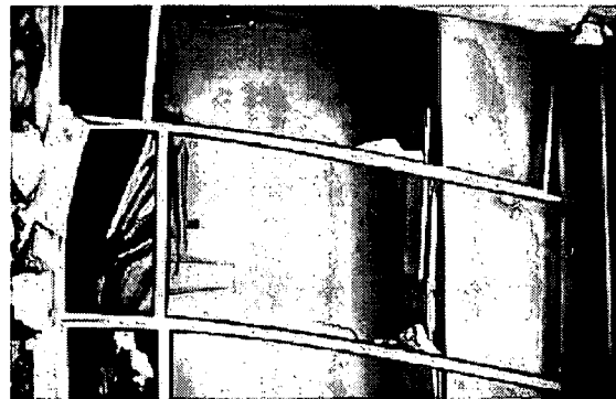
Figure 3. Broken windows, close-up view. A graphic example of the result of severe drift experienced by a concrete structure in the 1964 Alaska earthquake and the resulting failure of the glass panes (photo credit: EERI, John F. Meehan).
