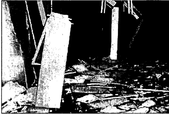
Figure 4. Fallen light fixture. These light fixtures, which were supported by the hung ceiling, fell when the ceiling distorted in the 1971 San Fernando Earthquake. The typical safety measure for fluorescent fixtures such as these is to attach back-up safety wires to them and anchor these wires to the floor or roof structure above, so that even if the ceiling grid distorts or collapses, the light fixture will not fall (Photo credit: EERI James L. Stratta).
