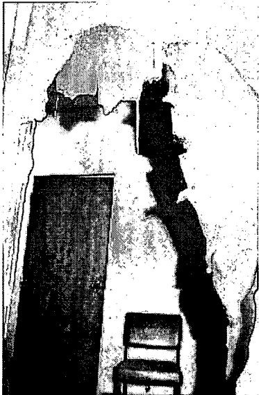
Figure 5. Escape hole made through partition and view of jammed door. In the 1979 Imperial County, California Earthquake, the door to this office in the imperial county services building was jammed shut by the distortion of the structure. The occupant was trapped until co-workers broke through the sheet-rock clad metal stud partition wall (Photo credit: EERI, Christopher Arnold).
